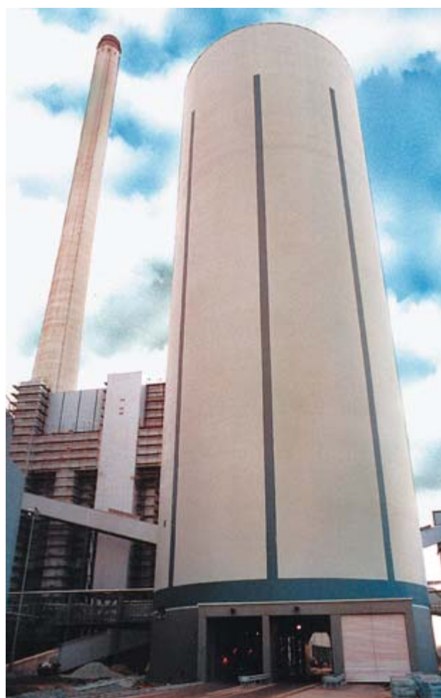
Claudius Peters - Duocell silo (31 m diameter) with truck loading facilities
