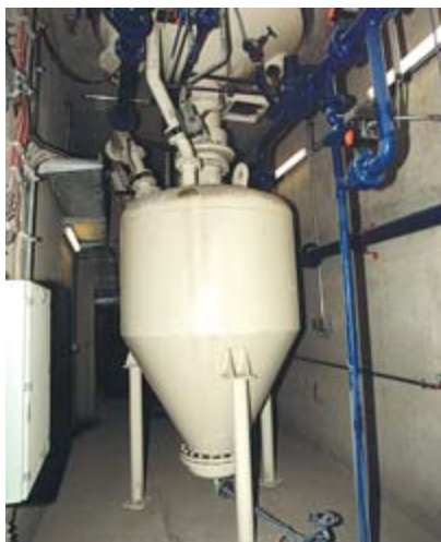
Ash transport pressure vessel
